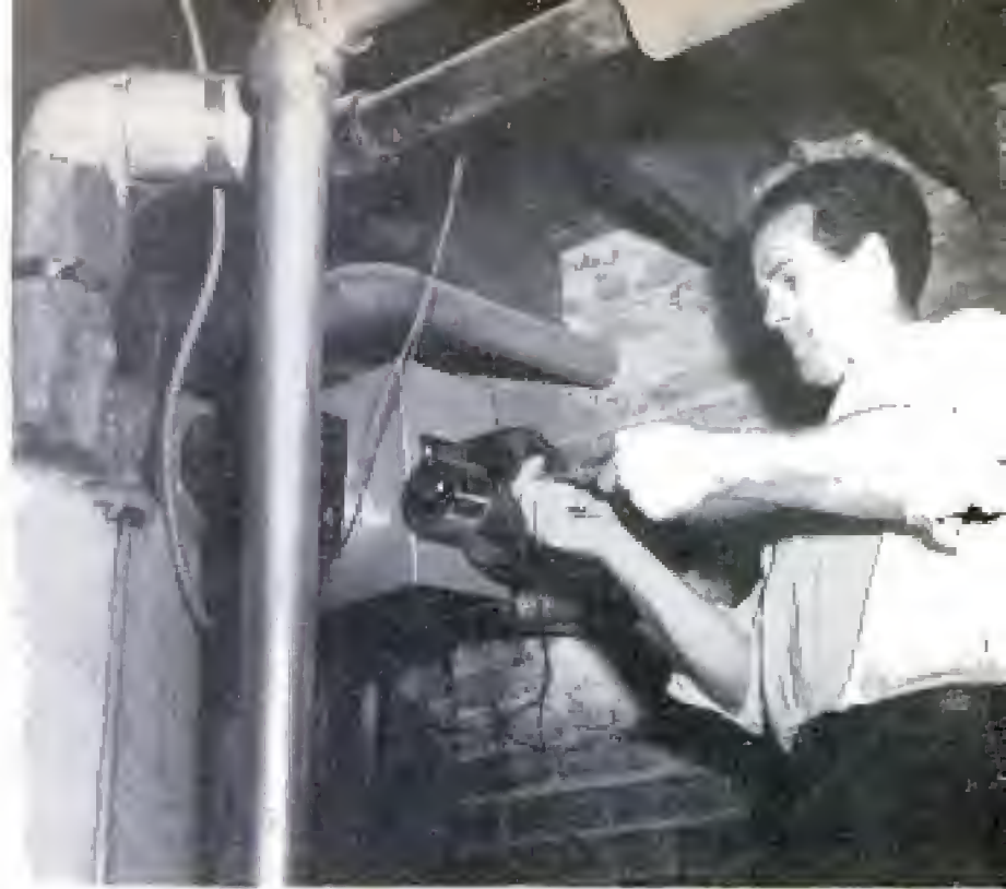
Above, the Free Heater can be installed in fairly limited space, either horizontally or vertically. Below, typical installation showing Free Heater, blower and thermostatic control for motor
